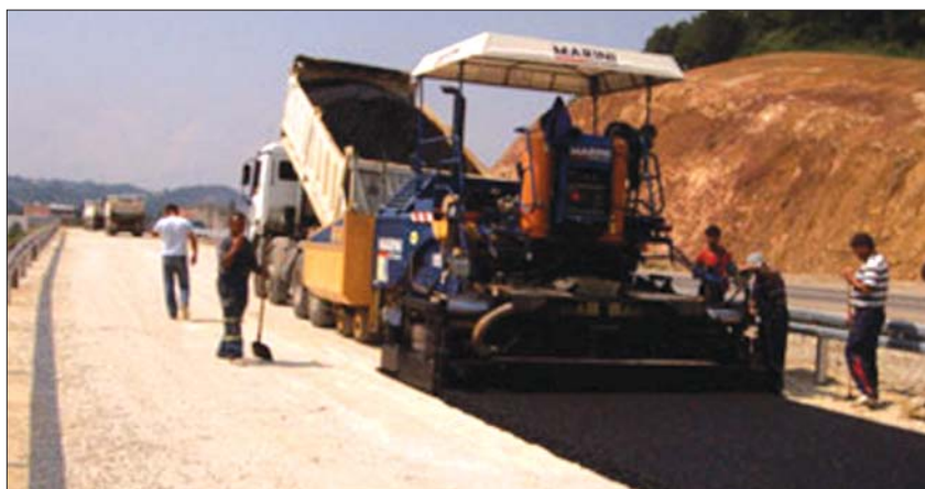
Dug put do autoceste u Banjoj Luci
